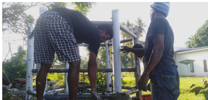
Gambar 5. Pengecoran rumpon Bio FAD's
