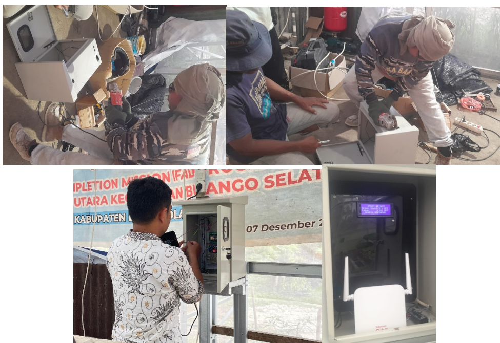
Gambar 7. Proses Pemasangan Smart Irrigation System Berbasis IoT
