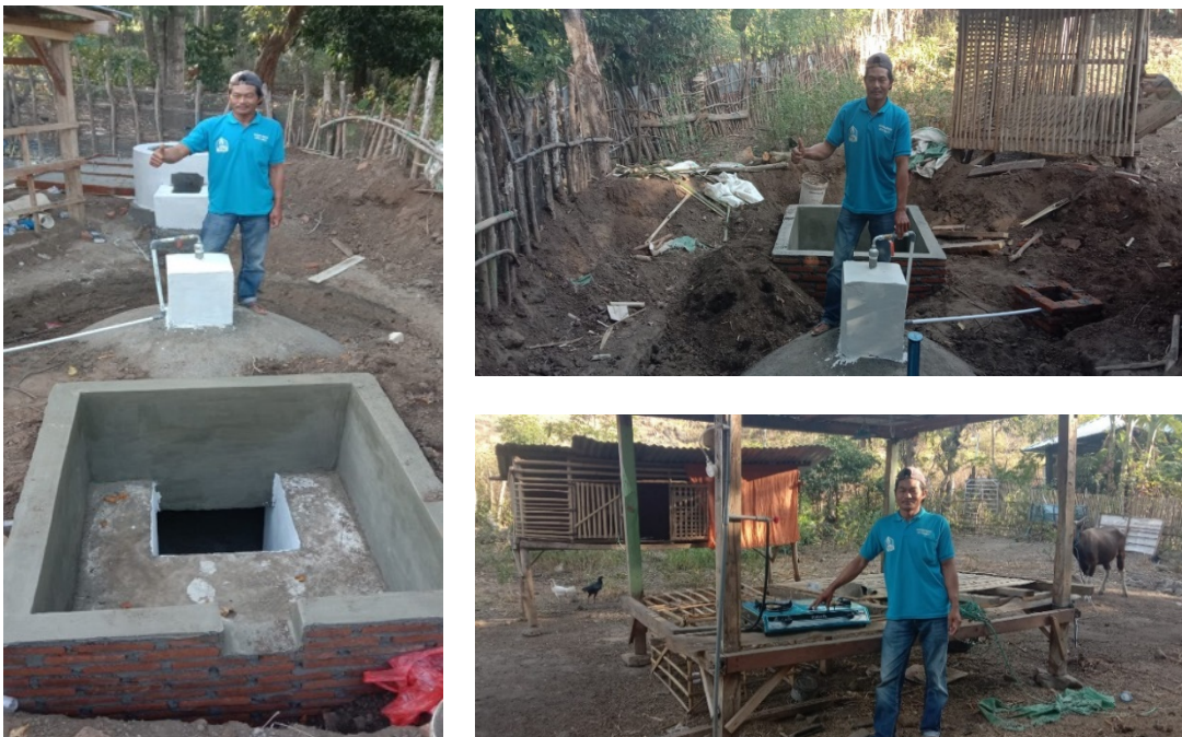
Gambar 4. Proses Instalasi Digester
