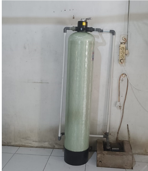
Gambar 5. Alat filter model backwash
